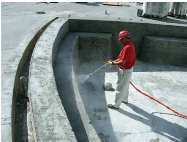
Applying sealer to pool on 14th floor condo
