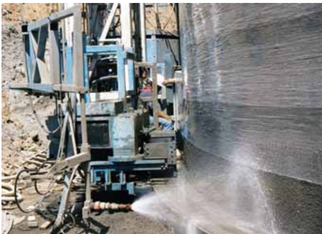
Fig. 7: Plastic wrapping of shotcrete cover coat for curing
