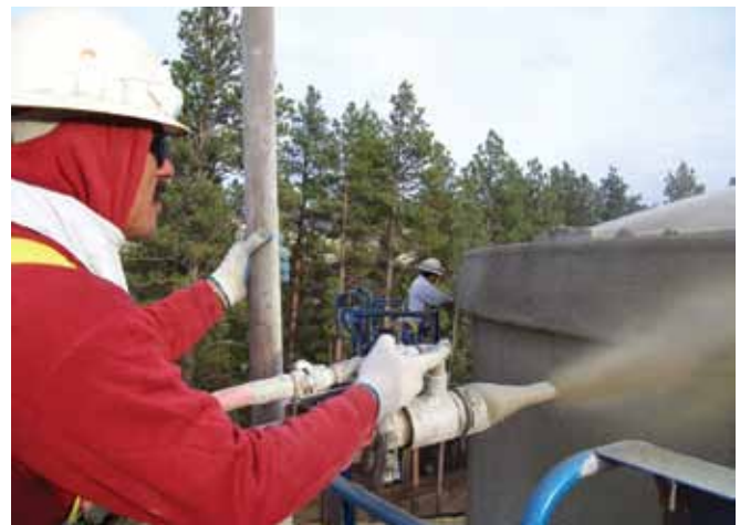
Fig. 9: Shotcreting dome ring
