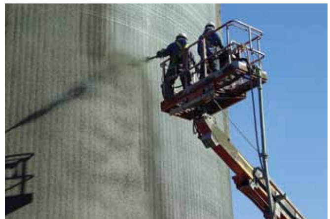
Fig. 3: Shotcreting of wrapped prestressing wires Photo courtesy of Natgun Corporation
