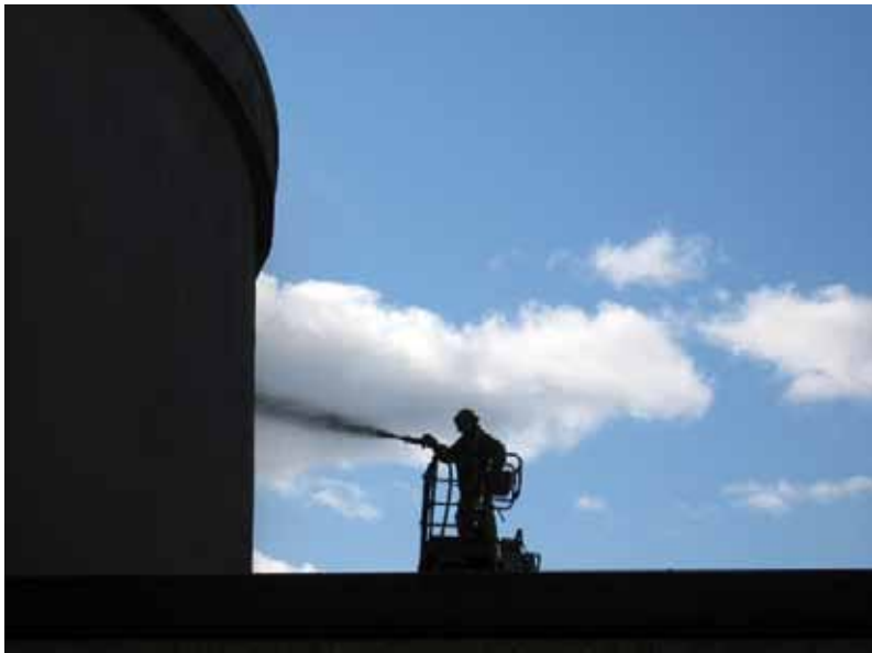
Fig. 10: Shotcreting final cover coat of a wrapped tank
