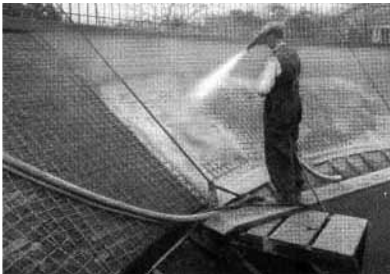
Fig. 1: Nozzleman applying gunite for a water storage facility in Pittsburgh, PA, 1919
