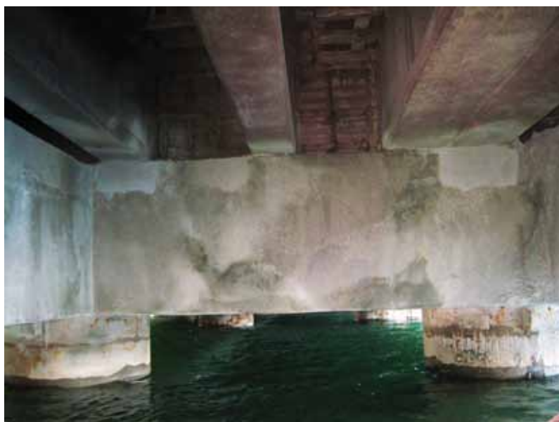
Finished repair zone beneath the wharf along some support beams
