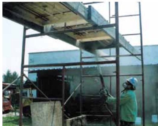
The gunning of an overhead panel during the certification
