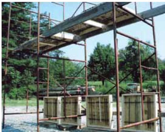
The scaffolding set up for both the overhead and vertical panels
