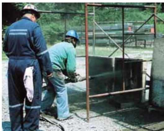
The gunning of a vertical panel with dry-process shotcrete
