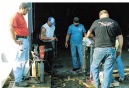
The core drilling of the shotcrete panels the day after gunning
