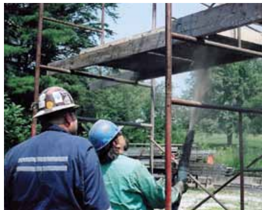
Nozzleman shooting his overhead shotcrete panel
