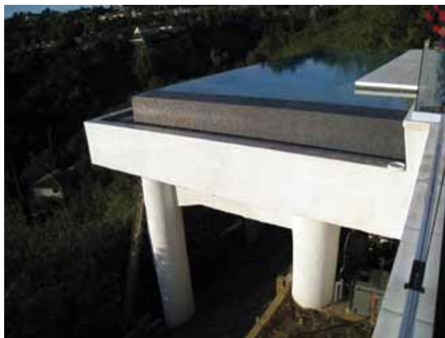
Pier-supported, out-of-grade swimming pool required complicated false work during construction
