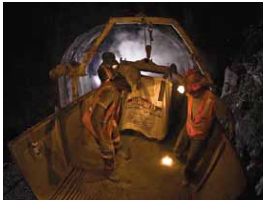
Workers on the Heartland Corridor project
