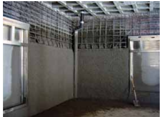
Lower portion of 18 ft (5.49 m) reinforced concrete wall
