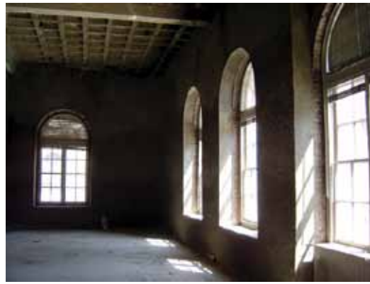
Internal corner with reinforced shotcrete around arched windows
