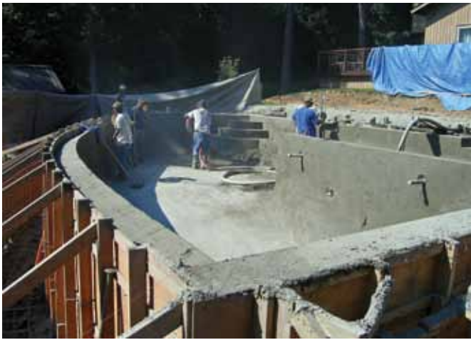
Main pool being shotcreted with tapered and curved negative edge
