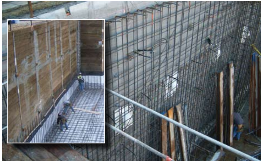
Fig 1: The Preprufe® SCS membrane (gray) is installed over the soldier piles and lagging (see insert). Preprufe® tieback covers (white) are installed over the wall's tie-back anchorages to ensure a continuous barrier. After the basement wall's reinforcing bars are installed, grout tubes are inserted through the bars and attached to the Preprufe® SCS membrane (photos courtesy of Johnson Western Gunite Company)
