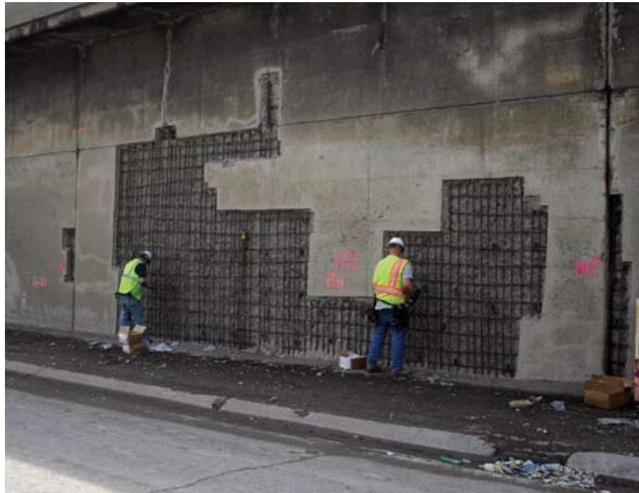
Securing reinforcing bar in chipped area prior to shooting
