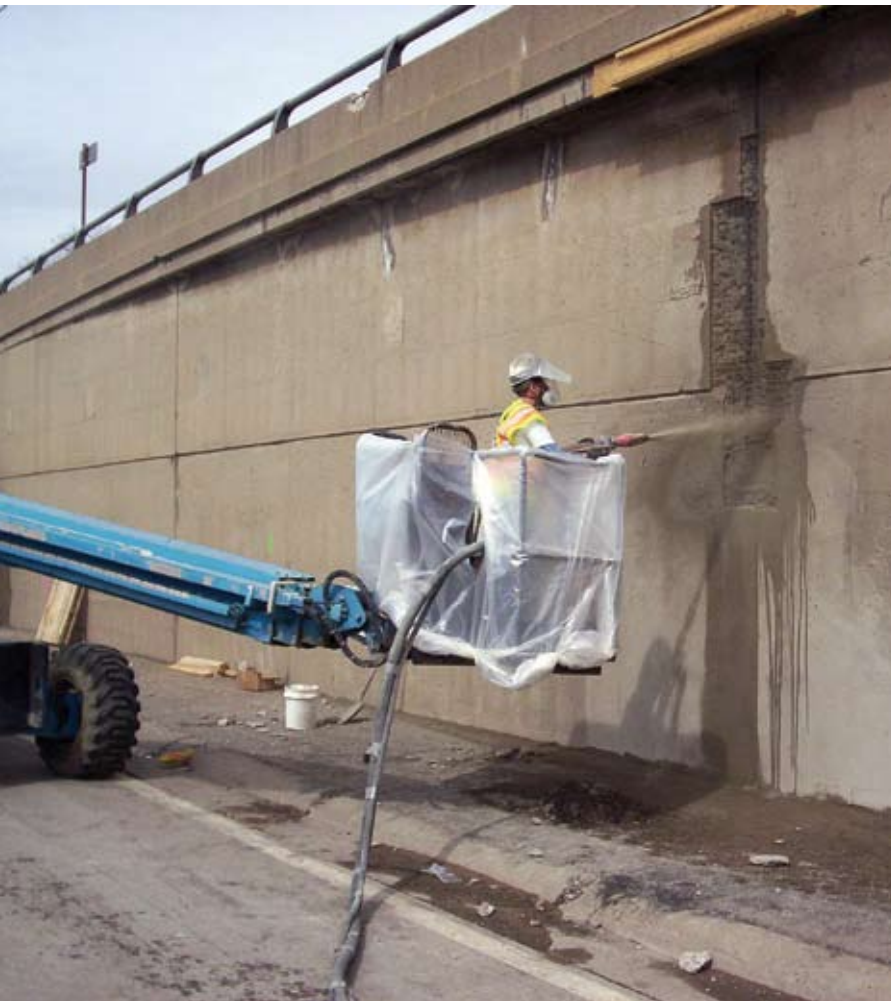
Shooting of elevated repair area
