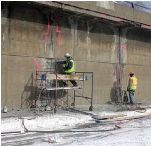
Removal of delaminated and spalling concrete with chipping hammers
