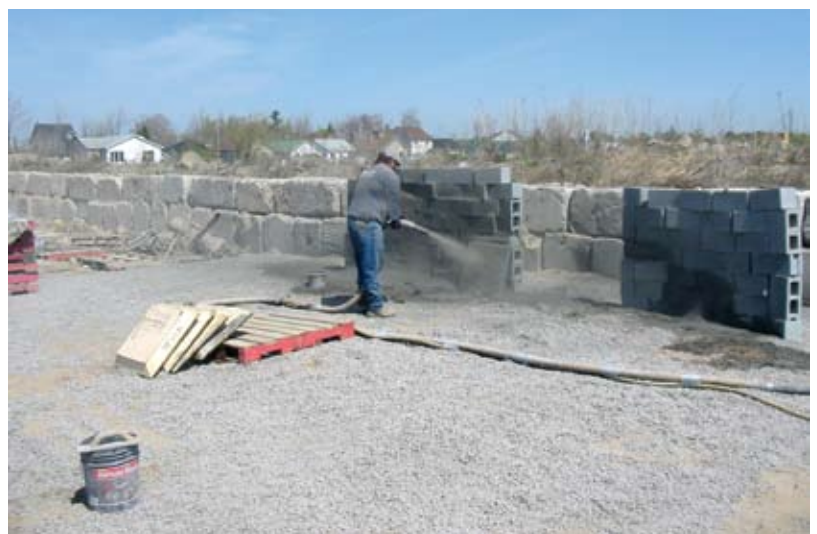
Fig. 1: ACI Certified Shotcrete Nozzleman—test panel shooting
