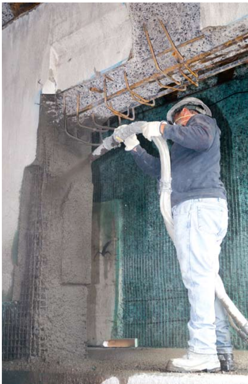
Fig. 2: City of Montreal—overpass shotcrete repair
