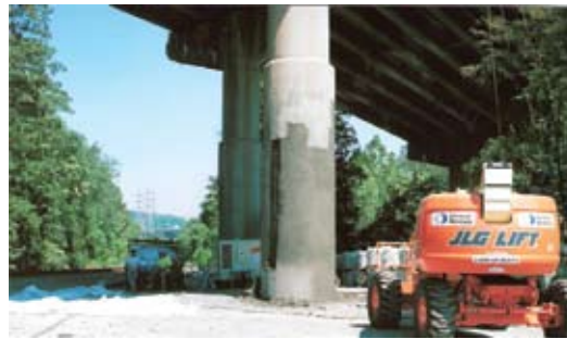
A shotcreted section of a bridge pier
