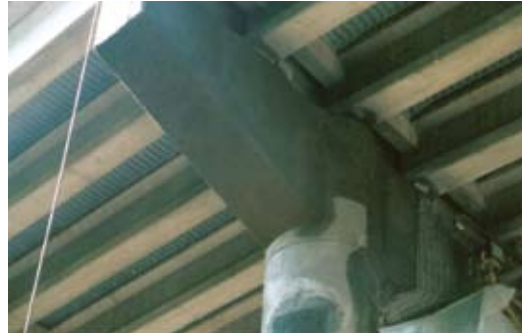
A completed shotcreted section of a pier hammerhead
