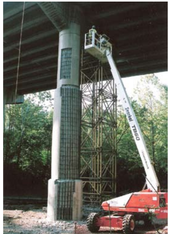
Concrete removal and surface preparation prior to the shotcrete placement
