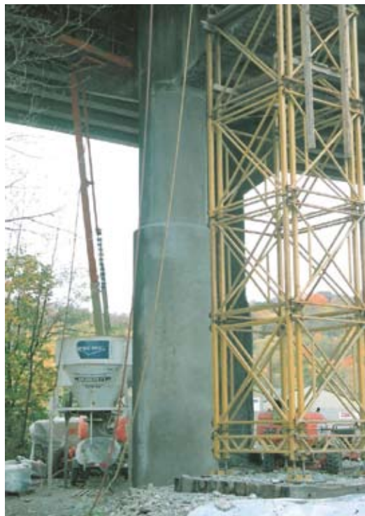
A completed shotcrete repair of a pier
