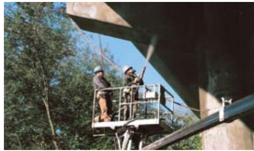
Overhead dry-mix shotcrete application to a pier hammerhead
