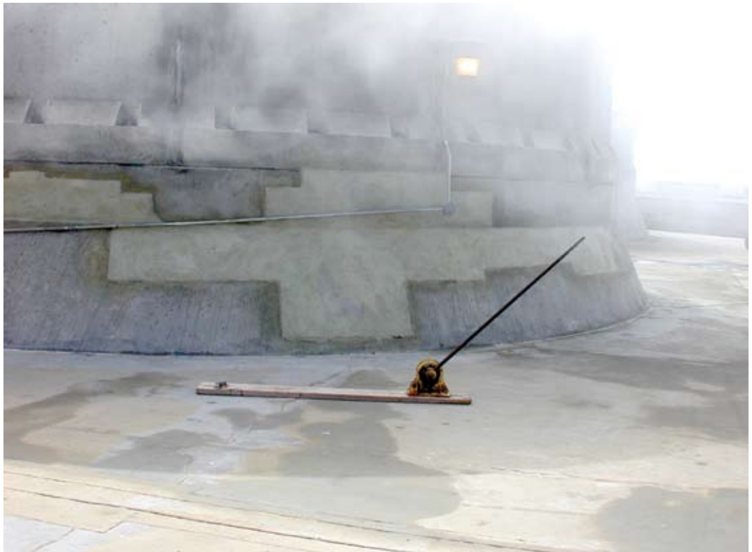
Project No. 3: Repaired fanstack assembly
