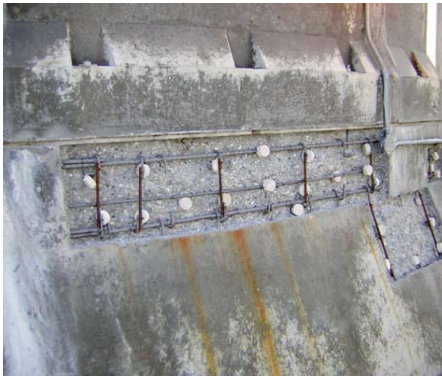
Project No. 2: Repair areas ready for shotcrete application
