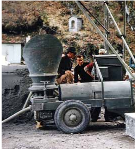
Fig. 4: American rotating-barrel gun (Jetcreter)
