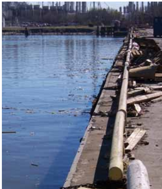
Typical state of the dock system prior to repairs
