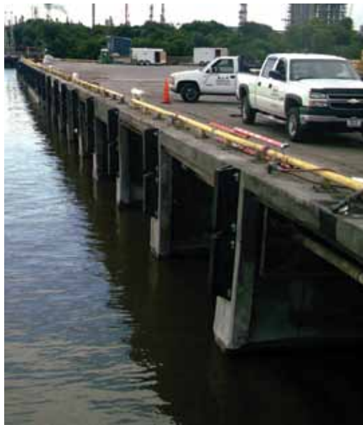
B & A Contractors, Inc., uses a bolted rubber bumper system to protect Manchester Terminals dock system from future damage resulting from ship strikes
