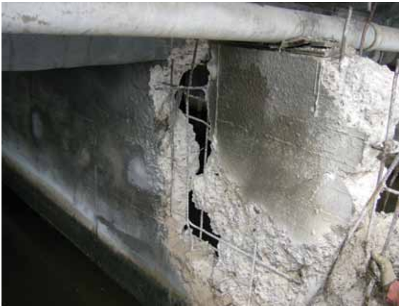
Using pneumatic tools, deteriorated concrete was removed, allowing for shotcrete repairs
