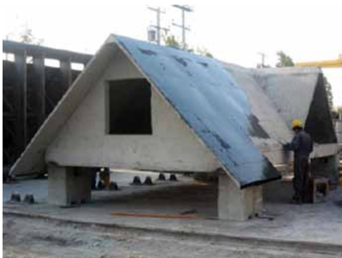
A Tekcrete™ roof module—a monolithic structure
