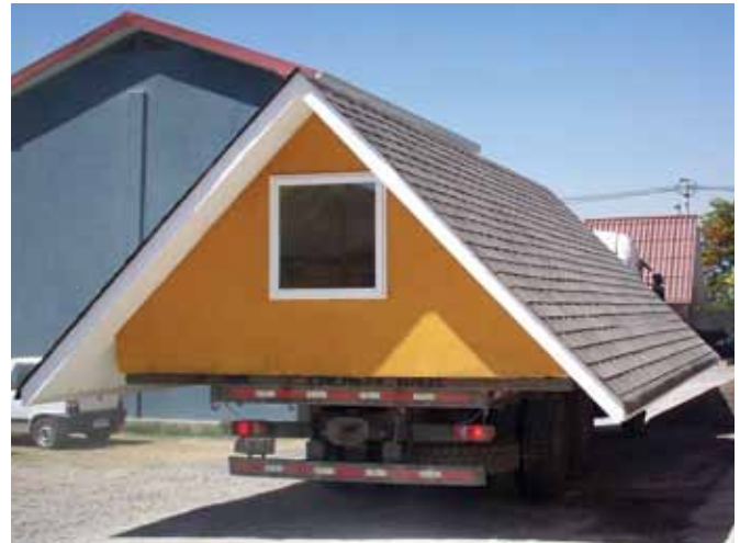
A fully finished Tekcrete roof module leaving the factory by flatbed truck
