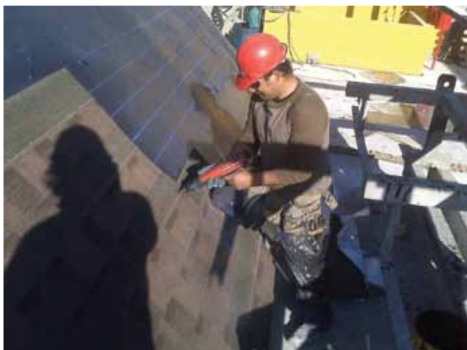
In-factory shingling of a Tekcrete roof module
