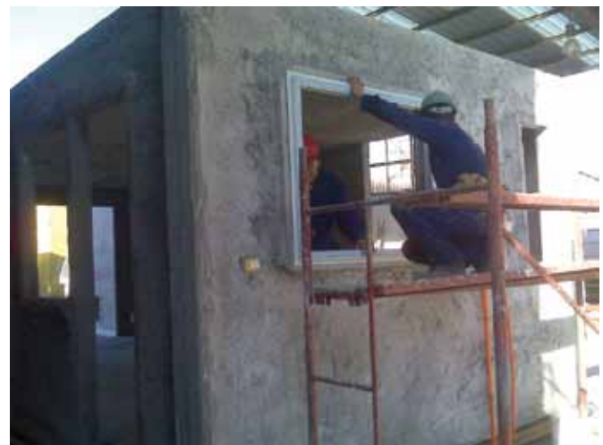
In-factory window installation on a Uni-Crete Cell housing module
