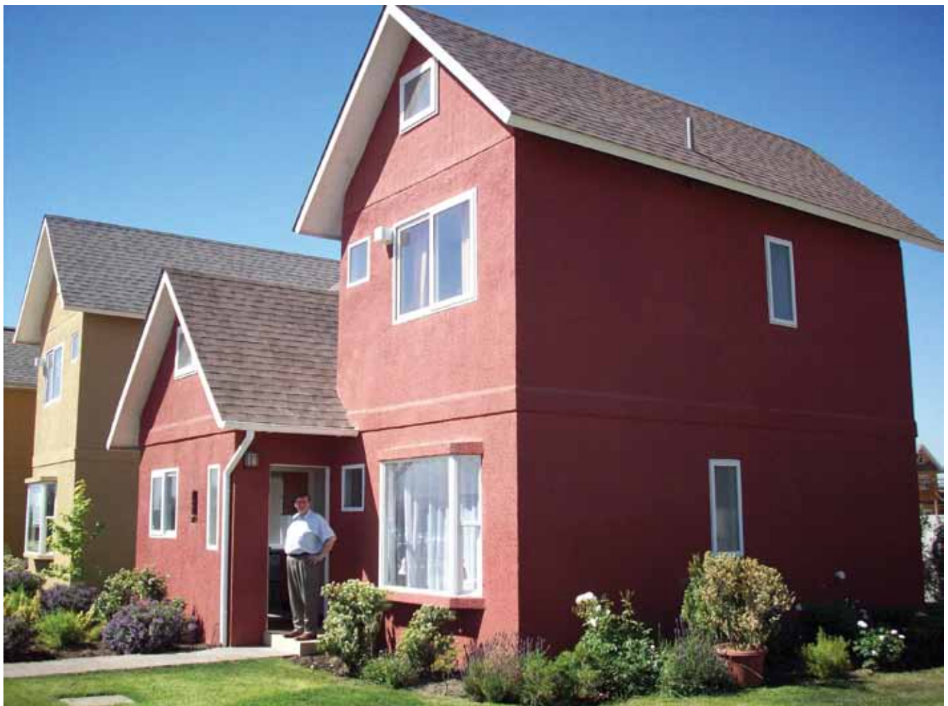
A fully finished Tekcrete home: seven modules, approximately 1125 ft 2 (105 m 2 )
