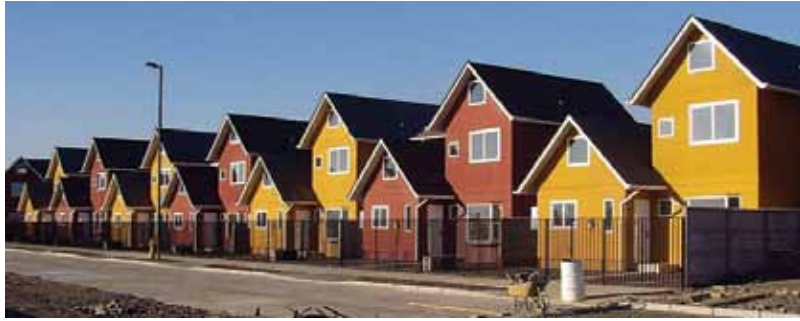
A line-up of Tekcrete homes in the Garden Valley (Jardines del Valle) Housing project
