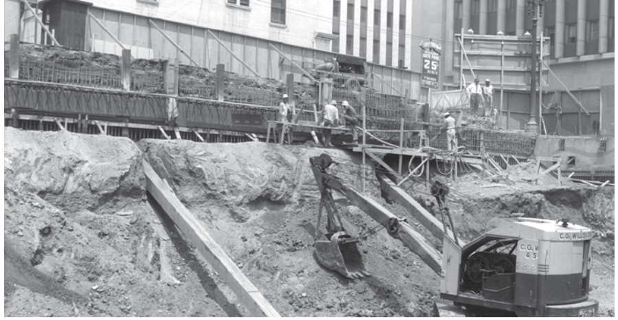
Gunitite shoring and basement wall project using dry-mix shotcrete, 1955
