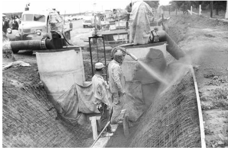
Canal lining project in southern California using dry-mix shotcrete, 1954
