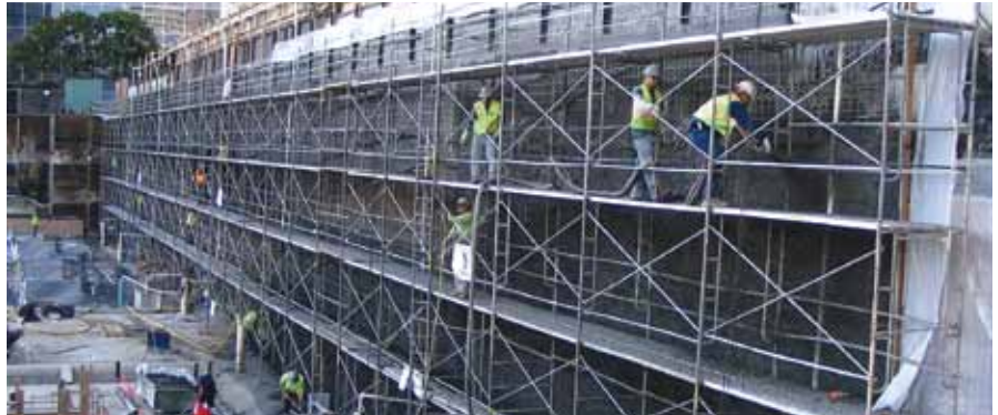
Gunitite shoring and basement wall project using wet-mix shotcrete, 2005
