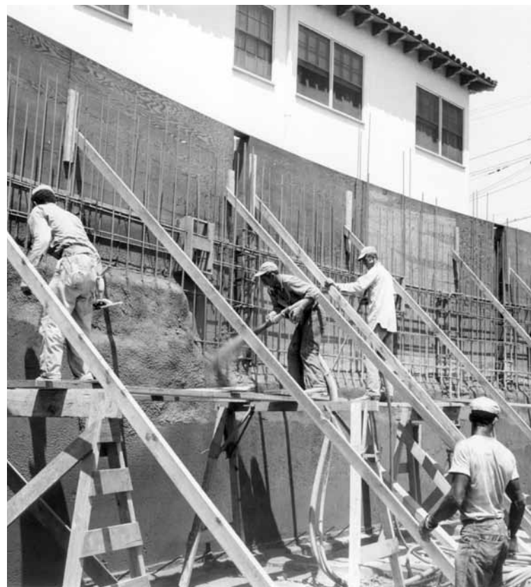
Structural retaining wall project using dry-mix shotcrete, 1955
