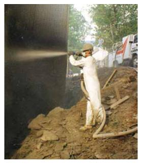
the same ball is thrown at the wall at a slower speed, the ball would still bounce off, but only a small portion of the paste would stick to the wall. The paste would not be forced into the pores of the wall. It would either strike the wall and fall to the ground or stay on the baseball.
