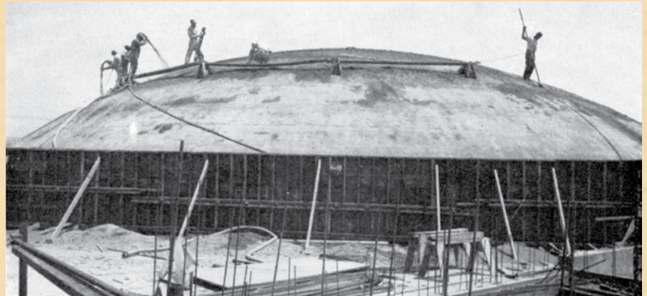
Guniting operation under way on the dome of White Memorial Seventh-Day Adventist Church. Height of dome above the floor is 70 ft; the diameter is 107 ft
