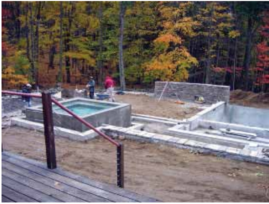
The pool and spa connected by the runnel system
