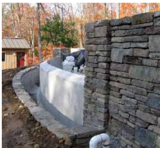
Catch basin for pool, with fieldstone veneer being applied
