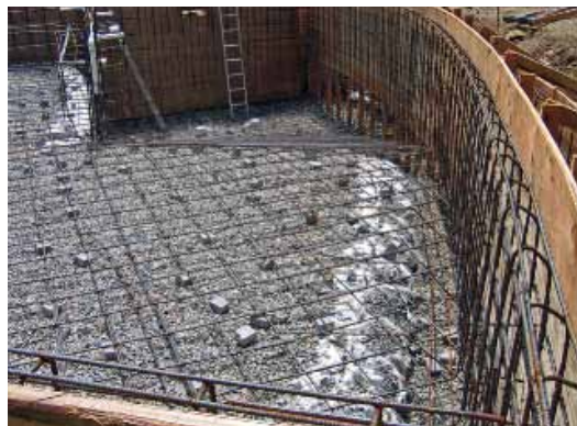
Negative edge pool—reinforcing steel being installed over the sloping floor profiles
