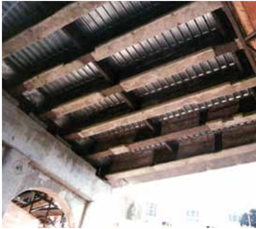
One of the spans after the damaged shotcrete was removed and the anchors and mesh were installed
