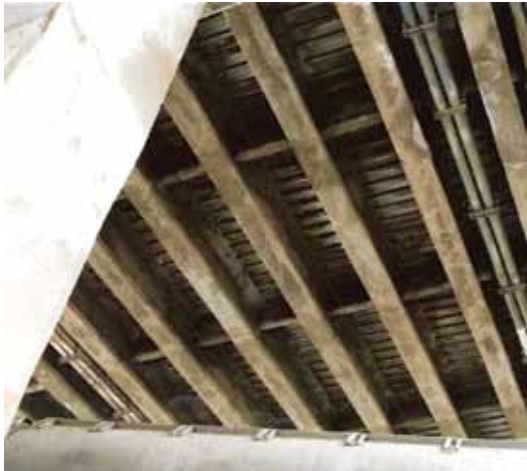
Bridge after repairs
