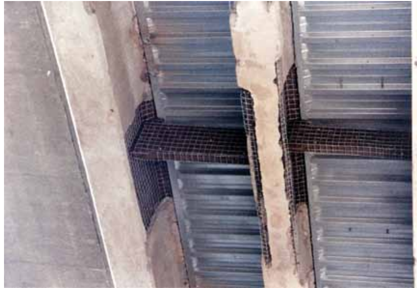
Close-up of the 41st Street Bridge connections
