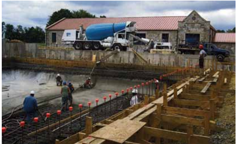
Floor construction joint
