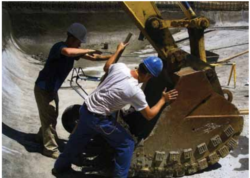
Removal of rebound and concrete trimmings
