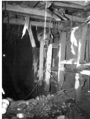
Fig. 13: Timber sets at Creighton Mine
