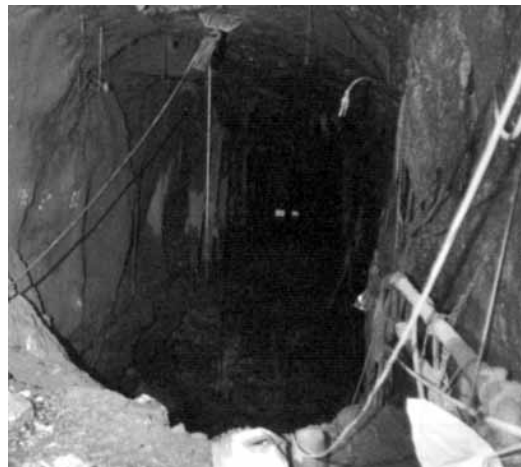
Fig. 14: Shotcrete use to replace timber sets
