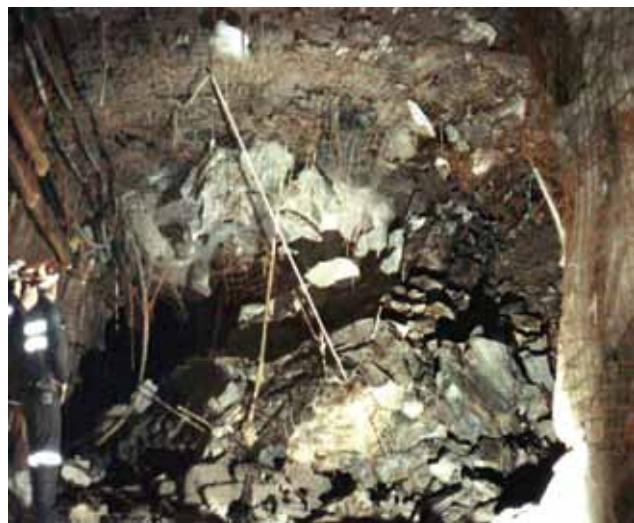
Fig. 7: Rock burst
