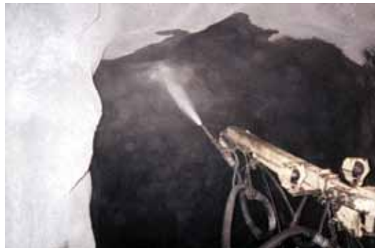
Fig. 9: Application of boltless SFRS
