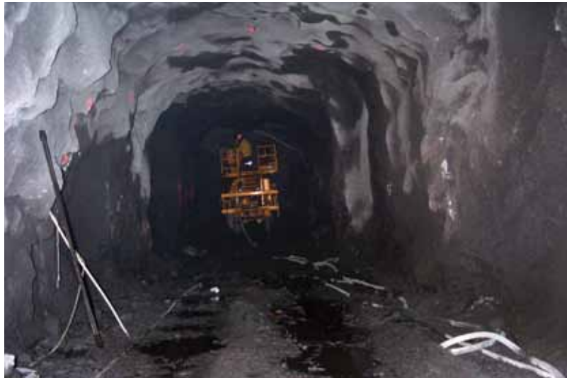
Fig. 10: Sublevel drill drift supported with boltless SFRS
