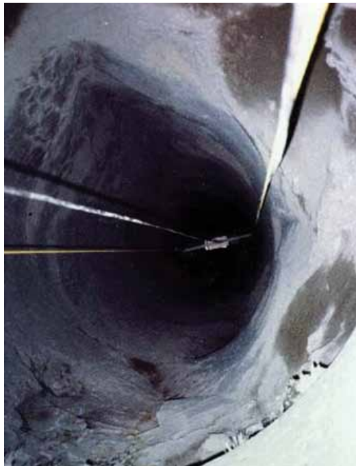
Fig. 2: Shotcrete use in raise
