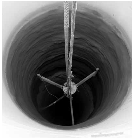
Fig. 6: Shaft lining using a robotic shotcrete rig
