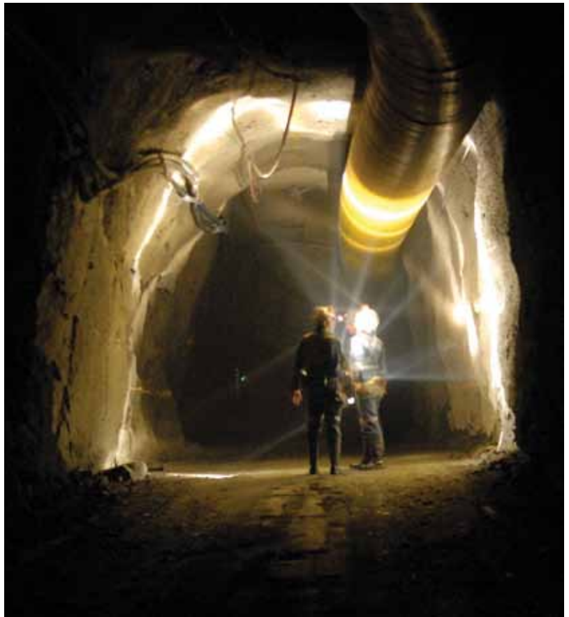
Fig. 1: Successful ground stabilization with FRS and bolts
