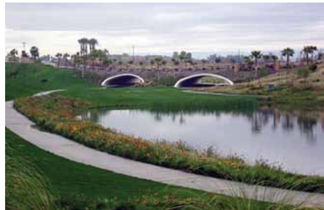
Bridge/culvert/golf cart tunnel combination at Shadow Hills in Indio, CA
