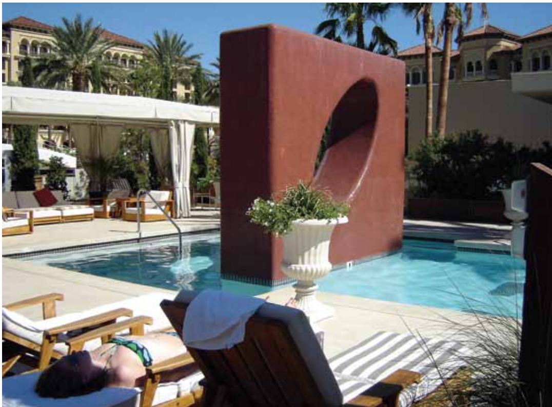
This monolithic structure is the main feature of the spa pool and cabana area at the Green Valley Ranch & Resort in Henderson, NV, and is made entirely out of shotcrete
