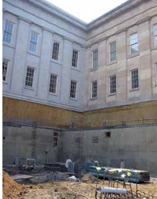
Smithsonian Patent Building below-grade wall retrofit project in Washington, DC
