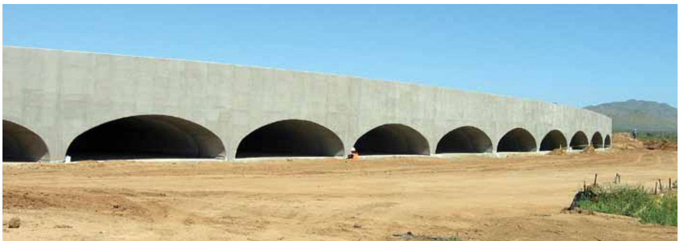
Vista Verde eight-barrel arch culvert in Rio Verde, AZ
