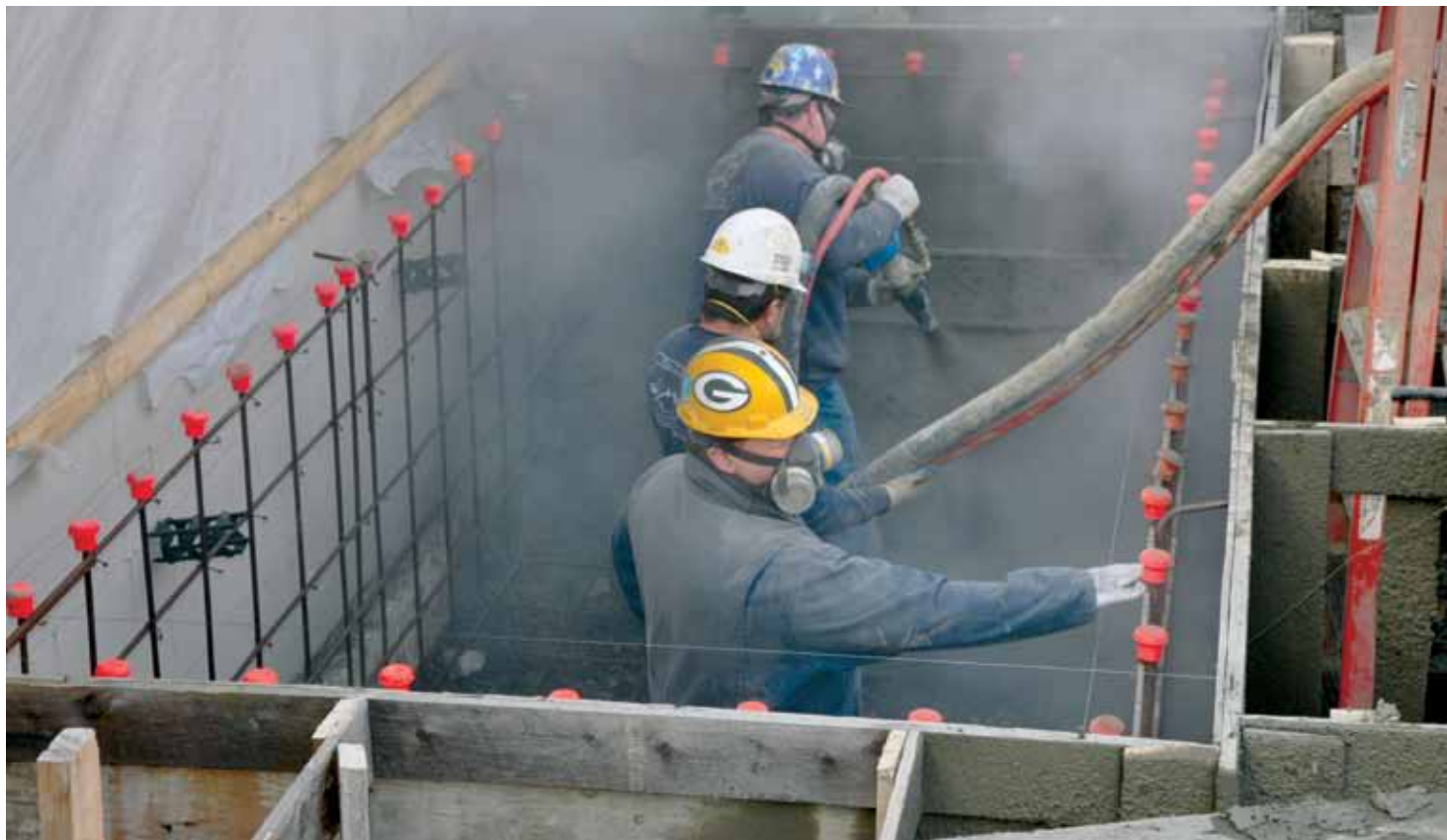
A watertight containment tank for off-road diesel tanks to be installed inside
