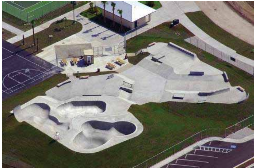
Overview of an 18,000 ft 2 (1672 m 2 ) skatepark in Englewood, FL
