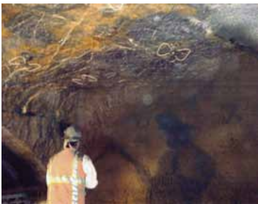
Shotcrete being applied to tunnel walls by ACI certified nozzleman
