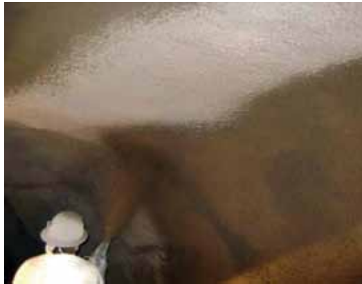
Lattice girder tunnel supports with final layers of fiber-reinforced shotcrete
