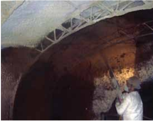
Placing initial layers of fiber-reinforced shotcrete
