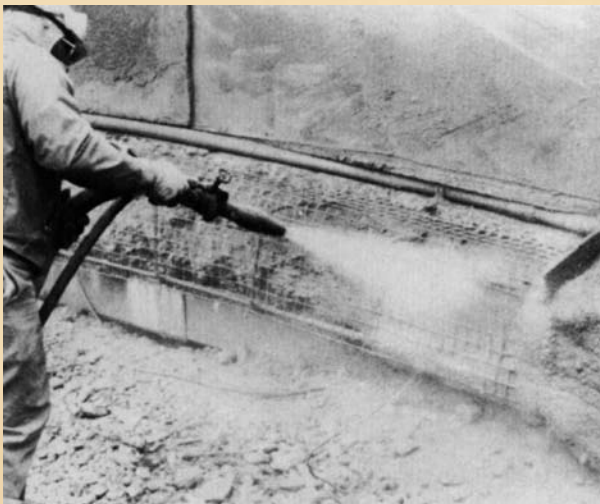
Shotcreting fascia beam; area to right is overshot
