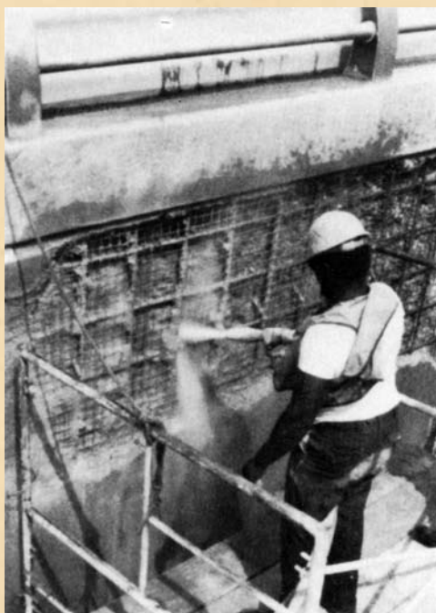
Wetting down an area prior to shotcreting
