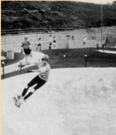
A skatepark constructed by using shotcrete
