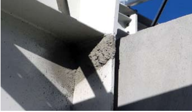
Looks like a small bird's nest but it is not. Unfortunately it is heavy overspray that will need to be removed
