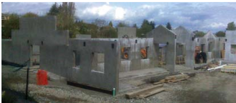
5000 ft 2 (465 m 2 ) of structural shotcrete walls
