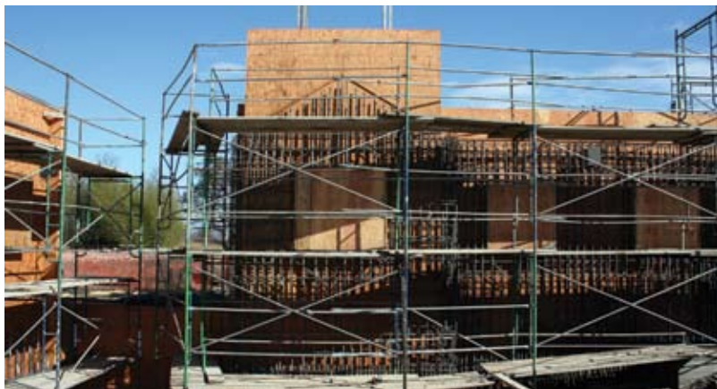
Difficult roof line and highly congested reinforcing steel
