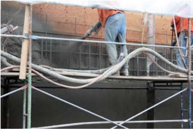
Bench gunning placement method
