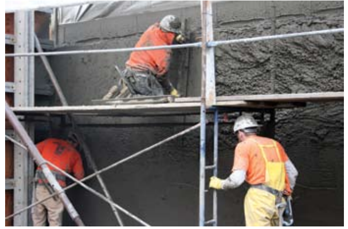
Cutting and finishing shotcrete wall
