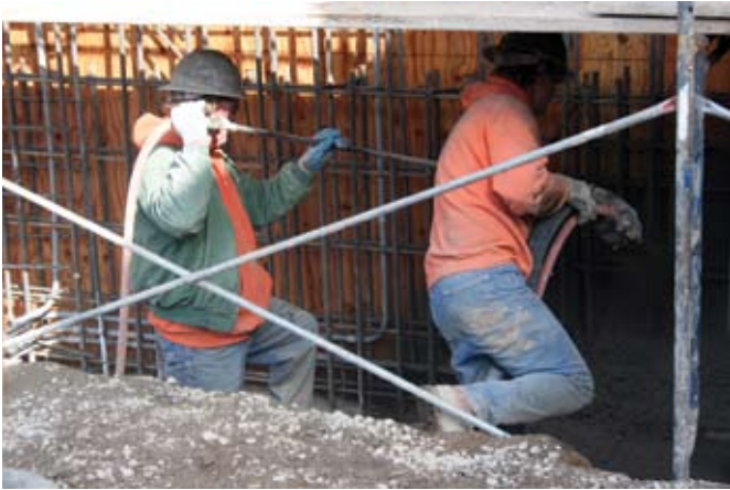
Bench gunning and blow-pipe operator
