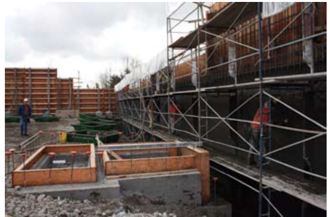
Rodding and finishing the wall
