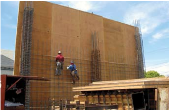
Reinforcing bar being installed after form is secured with chamfers on form for architectural design
