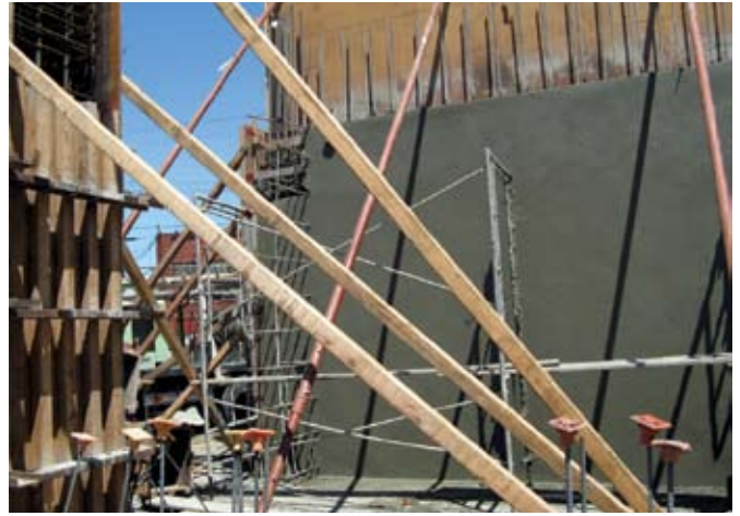
Completed high walls and the sand float finish
