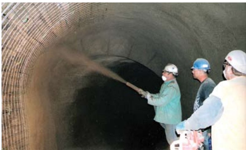
Dry-shotcrete process job under Route 51 in Aliquippa, PA, in 2006
