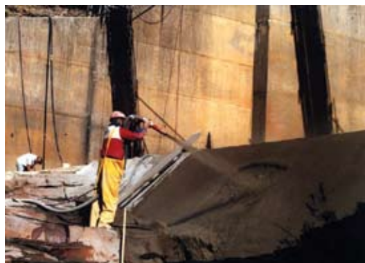
Dry-shotcrete installation at base of Two Lick Dam in Indiana, PA
