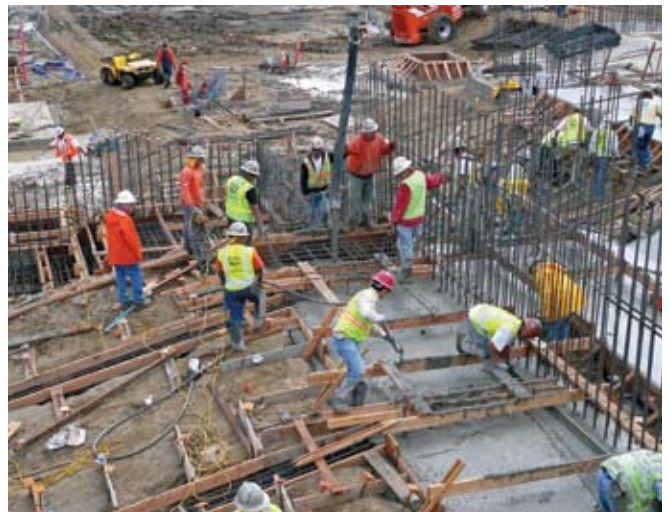
Placing concrete in a congested area after safety practices were implemented
