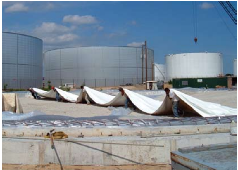
Air form being rolled out
