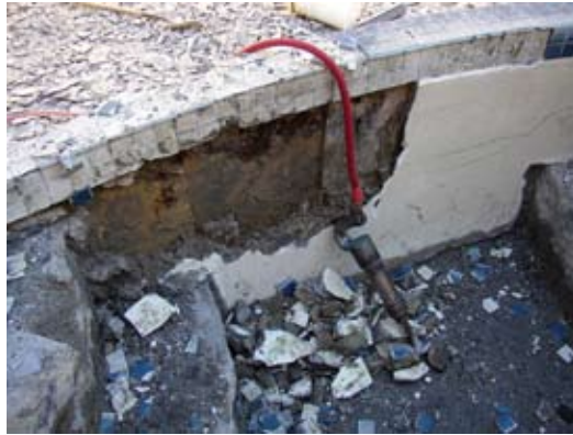
Fig. 10: It's not uncommon to find drywall left between the inner and outer layer of shotcrete when spa walls are taken apart for repair
