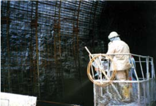
Figure 4: Shotcrete being applied to the canopy support structure
