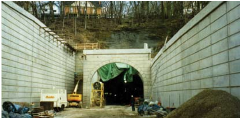
Figure 1: Tunnel portal and retaining walls
