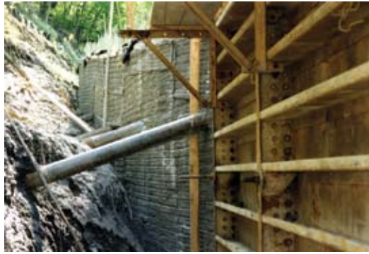
Figure 5: Backside of retaining wall using Stay-form and modular forms
