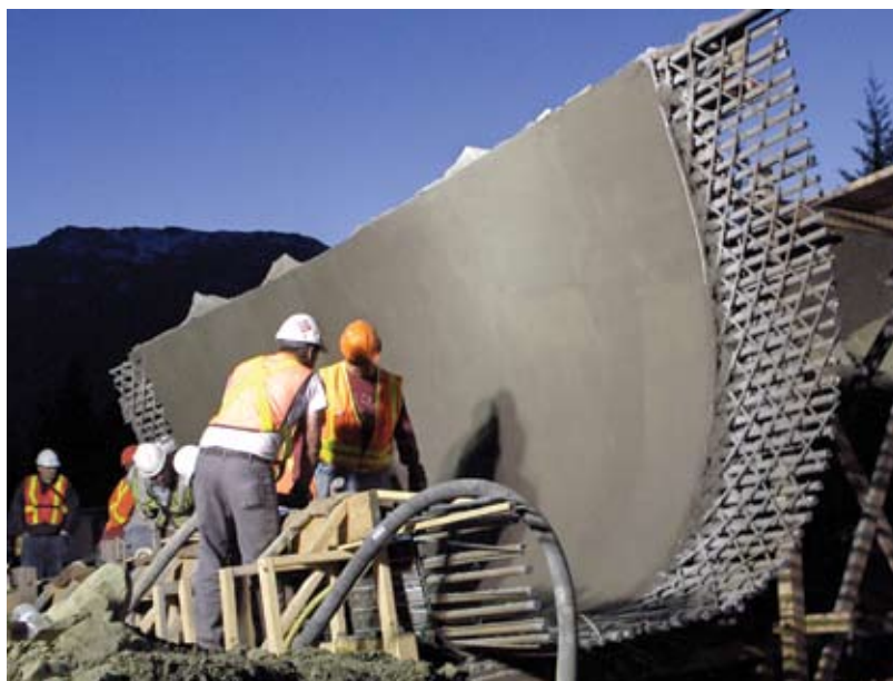
Fig. 3: Crew constructing mock-up on May 1, 2007
