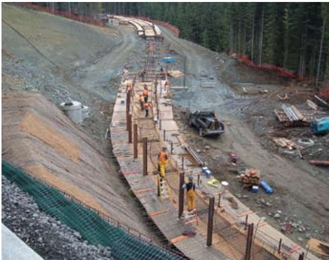
Fig. 5: Refrigeration piping being installed on jig assemblies
