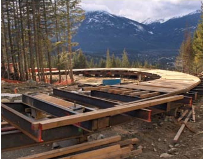
Fig. 4: Structural steel falsework system and base forms being installed
