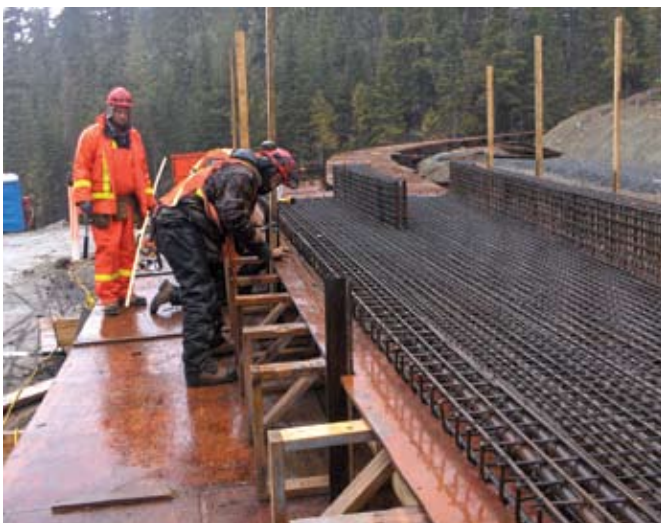
Fig. 6: Reinforcing bar installation
