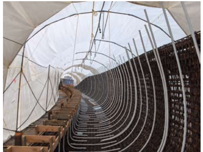
Fig. 8: Tents, lights, and sprinkler system installed—section ready for shotcrete
