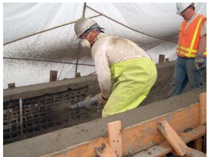
Fig. 9: Shotcrete being applied under the watchful eye of David Baranowski (VBFA)
