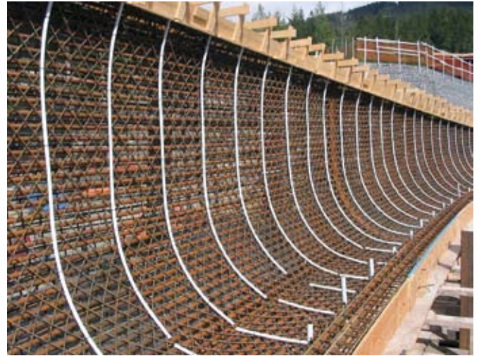
Fig. 7: Formwork and finishing screeds (plastic pipes) installed
