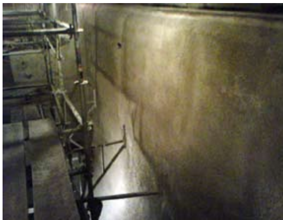
Completed opposite wall section of the ash hopper relined, October 2007
