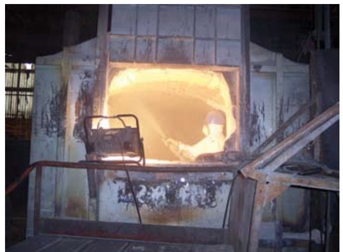
Shotcrete in aluminum industry (furnace)
