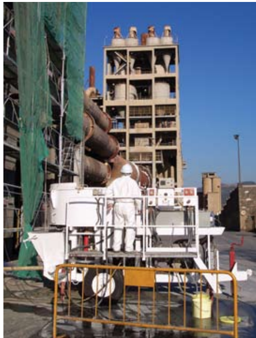
Shotcrete in cement industry (preheater)
