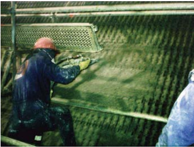
Shotcrete in power plant (boiler)
