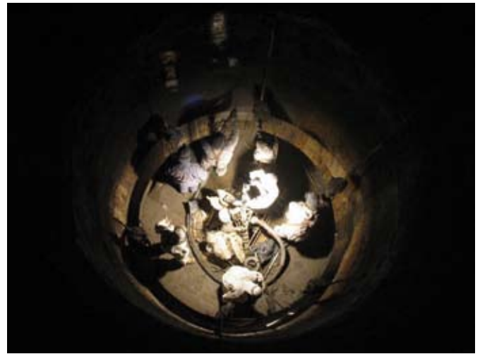
Shotcrete in petrochemical industry (chimney)
