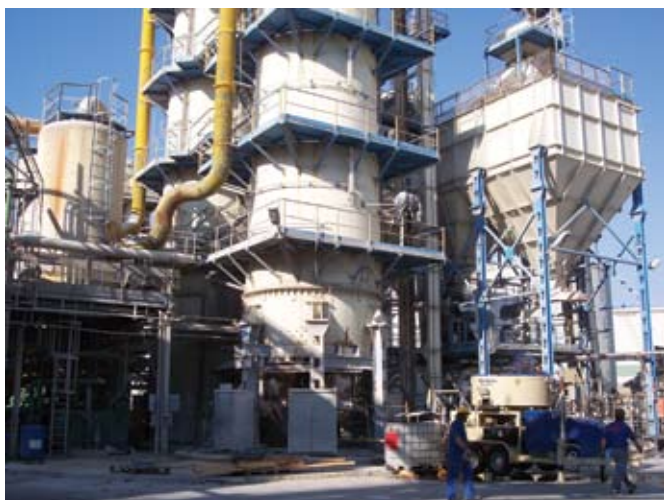
Shotcrete in lime industry (kiln)
