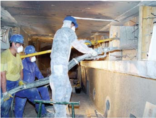
Shotcrete in steel plant (reheat furnace)
