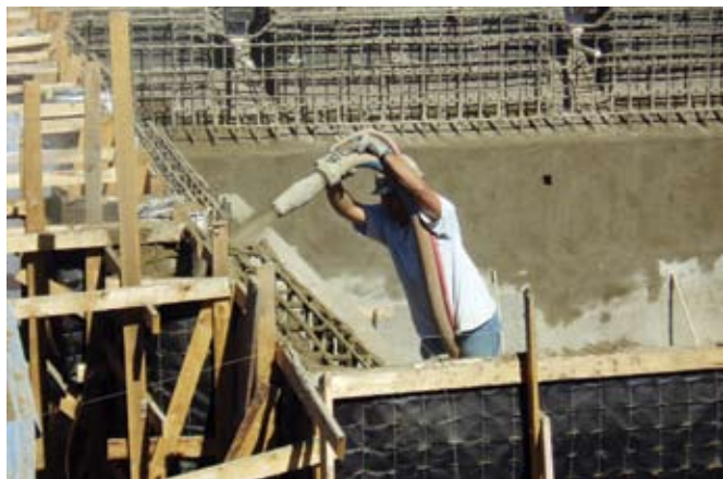
Dry-mix shotcrete application by an ACI certified nozzleman
