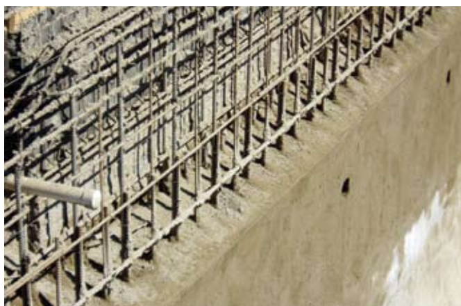
Awaiting next application in shotcrete process
