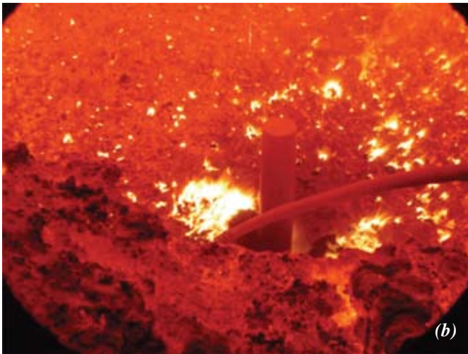
Fig. 4: Tap hole sleeve changing: (a) pumping equipment is placed near BOF mouth; (b) hot shotcreting R2U MgO-C castable for sleeve repairing; and (c) repaired region after shotcreting
