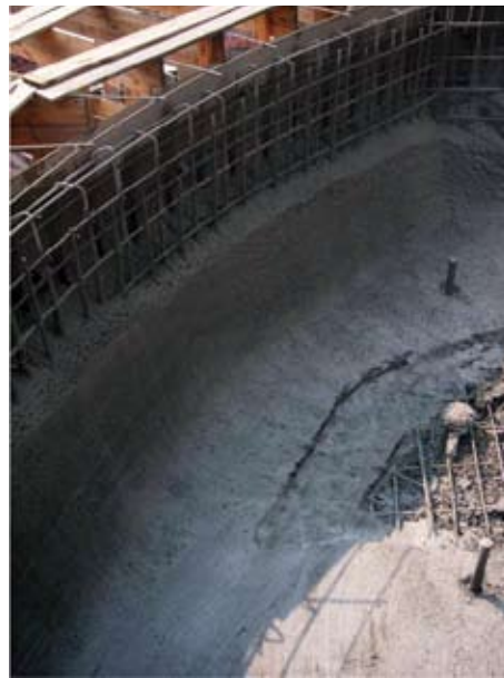
4000 psi (28 MPa) shotcrete installed concrete
