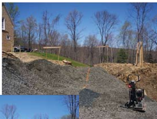
Removal of fill and installation of process material compacted in 6 in. (152 mm) lifts. Top of forms is the water height
