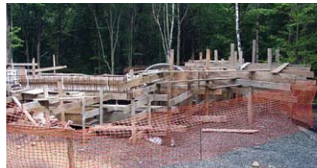
Rigid forming: 1 x 6 in. (24 x 152 mm) rough-sawn lumber with 1/2 in. (13 mm) steel and 6 in. (152 mm) on center
