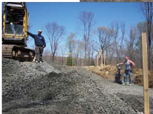
Removal of fill and installation of process material compacted in 6 in. (152 mm) lifts. Top of forms is the water height
