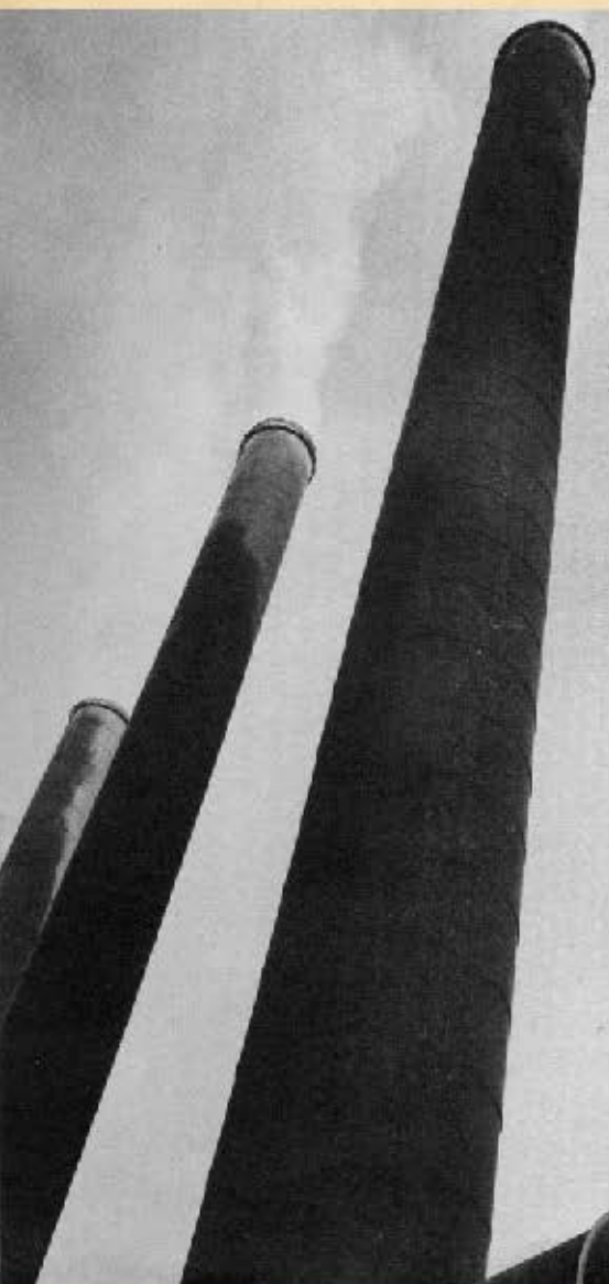
Fig. 4: Three power-plant stacks, lined with corrosion-resistant concrete. First stack lined in 1941, second in 1943, and third in 1945
