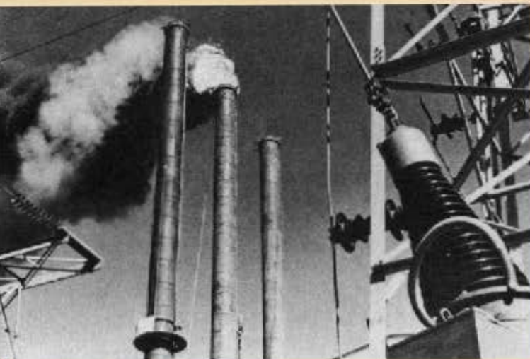
Fig. 3: Three 200-ft stacks at power plant burning acid sludge from oil refineries. Insulating, corrosion-resistant concrete linings protect steel under unusually severe conditions
