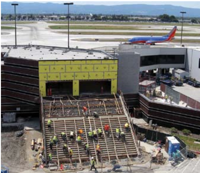
Terminal building emergency exit stairs
