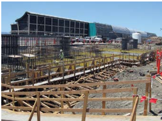
Large wall pile cap (1683 yd [1500 m] of concrete)
