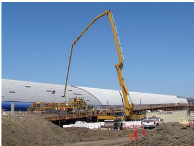
Pumping concrete on airport bridge
