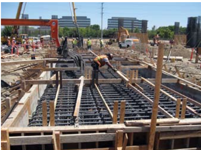
Wall pile cap before concrete placement
