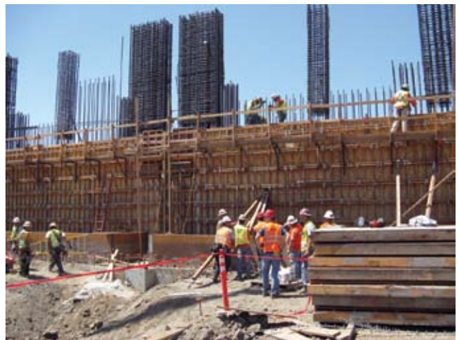
Shear wall forms
