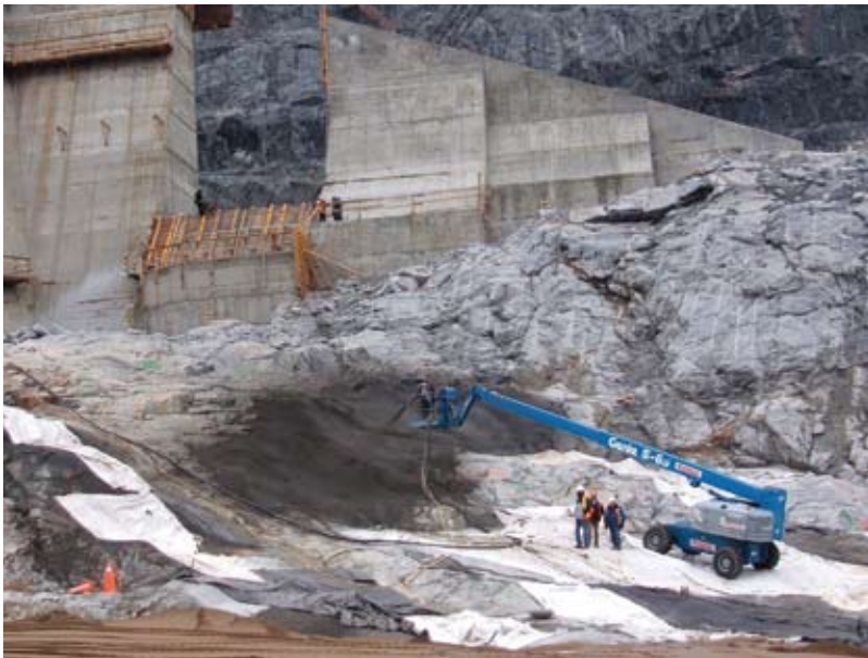
Fig. 4: Wet-mix shotcrete material application on the rock
