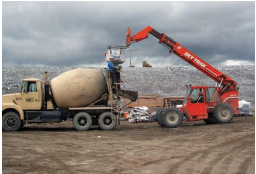
Fig. 2: Wet-mix shotcrete material production from bulk bag into a concrete truck
