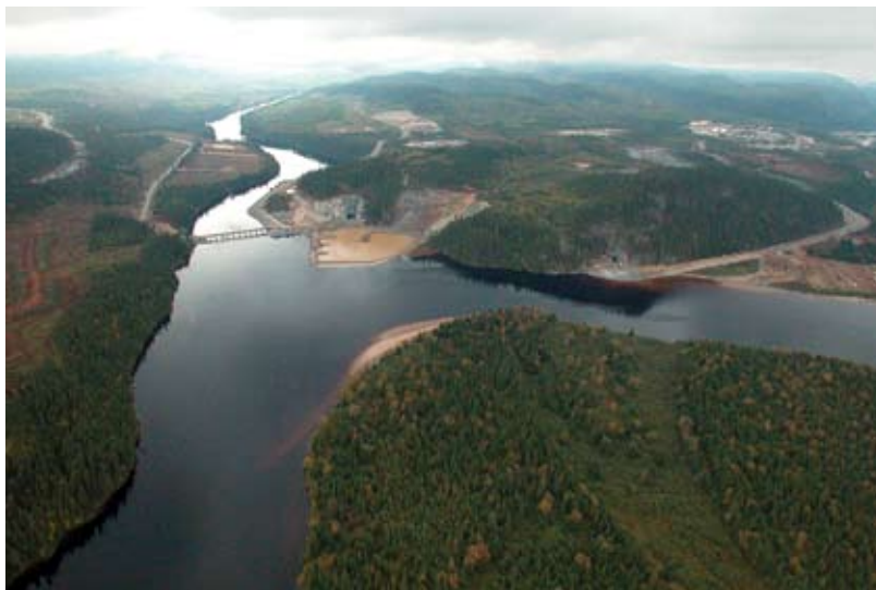
Fig. 1: General view of the project on the Péribonka River, September 2004 (Photo courtesy of Hydro-Québec)
