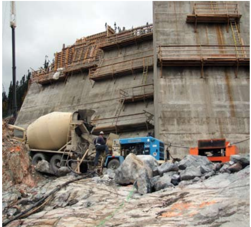
Fig. 3: Wet-mix shotcrete material discharge from the concrete truck into the pump
