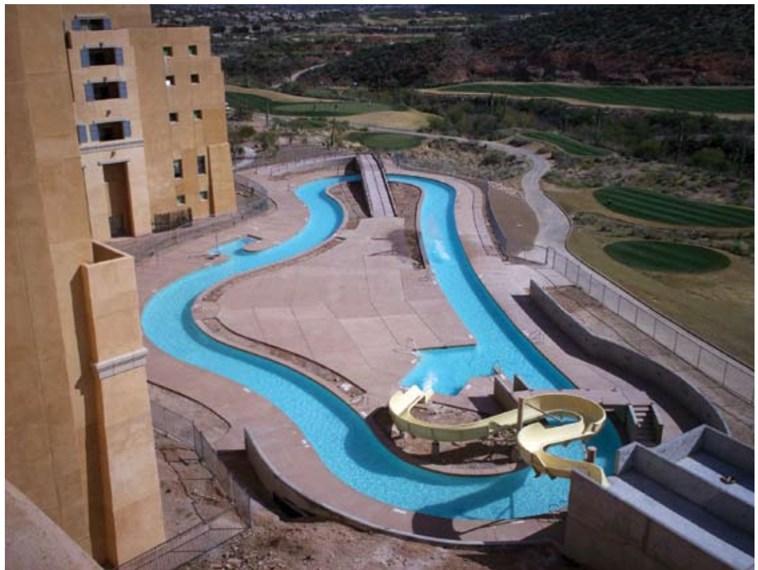
The lazy river close to completion
