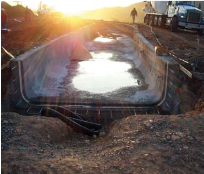
Shotcrete section adjacent to the unexcavated final section
