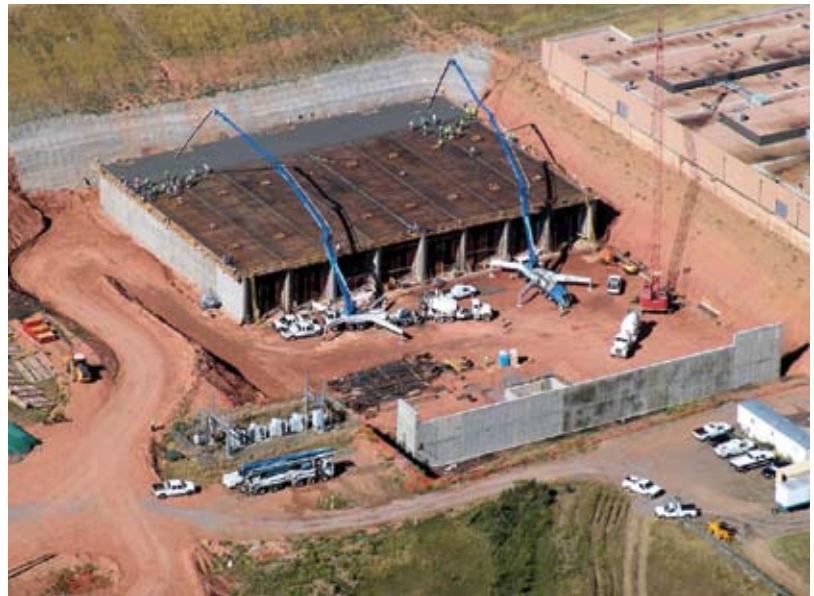
Shoring for expansion of water treatment plant
