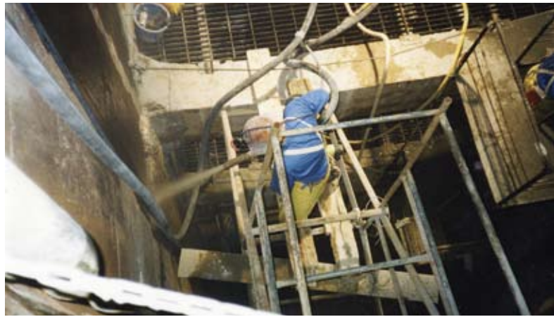
Dry shotcrete at pump station in Israel
