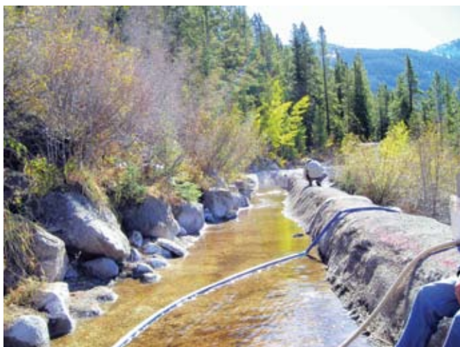
Lily pad diversion structure
