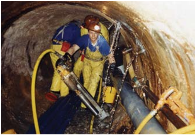
Tunnel repair at pump station in Israel
