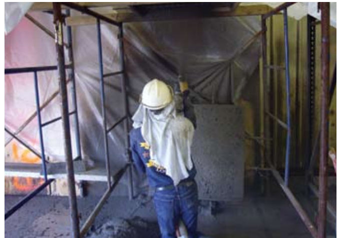
A shotcrete nozzleman certification test section
