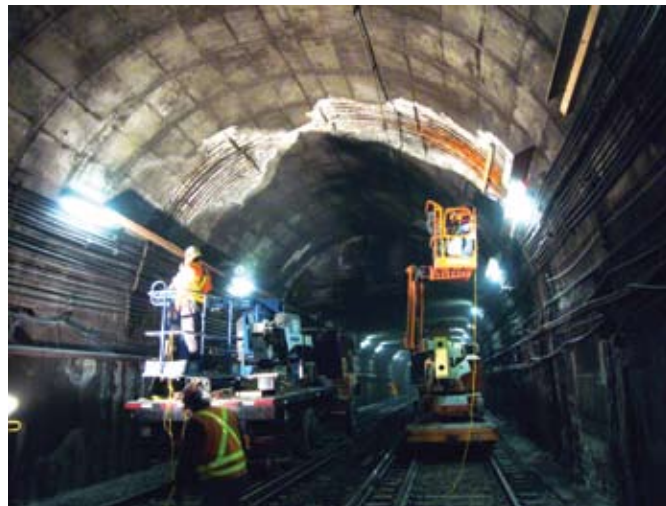
High-rail equipment during removal of delaminations
