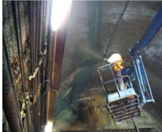
Applying shotcrete to tunnel arch
