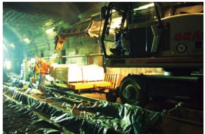
Shotcrete being unloaded from railcars at shotcrete machine
