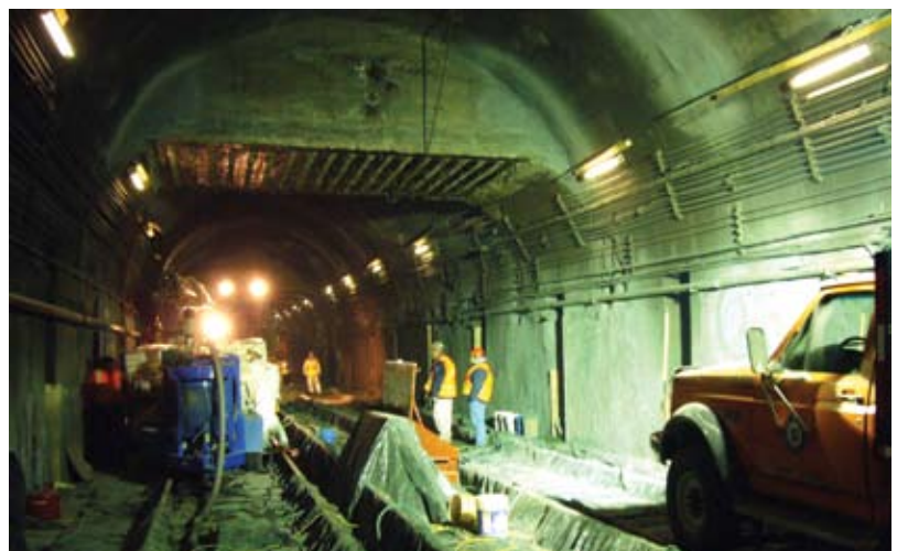
Completed shotcrete placement on walls and arch
