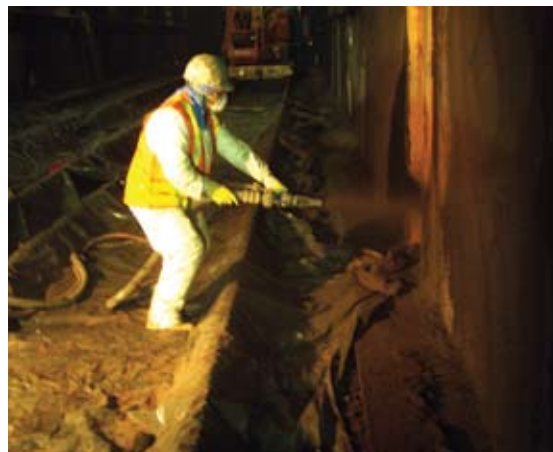
Applying shotcrete to tunnel walls
