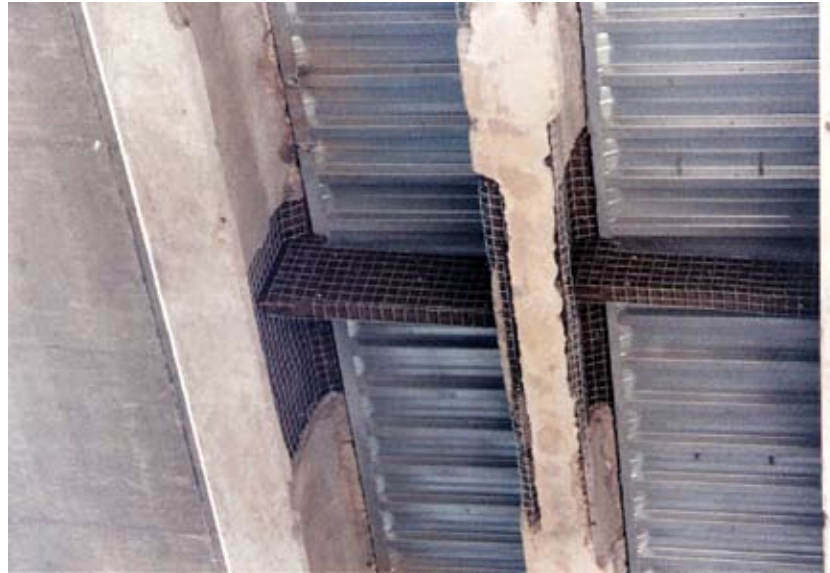
Close-up of the 41st Street Bridge connections
