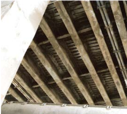
Bridge after repairs
