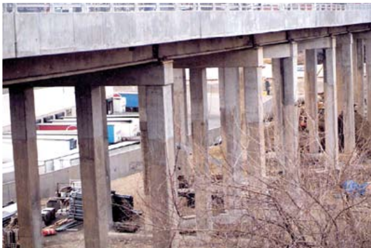
Piers on the east end of the bridge
